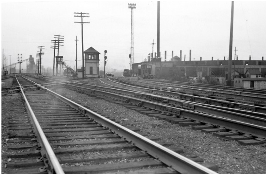
View looking eastward at Grandview Tower, where the Big Four double track main toward Cincinnati (foreground) crossed the single-track T&OC main toward Toledo diagonally at the two diamonds. Curving interchange tracks are just to the right and left of the diamonds. The west throat of the T&OC West Columbus Yard is just beyond Grandview Avenue, where a vehicle can be seen crossing. The small tower to the left is for a crossing guard. West Columbus Roundhouse is to the right. Photo circa 1940 from E Miller/BJ Kern collection, as shown on Columbus Railroads.
