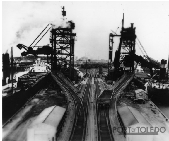
Rail car dumper facilities, Toledo, 1940s. National Museum of the Great Lakes: https://nmgl.org/coal-dumpers-lakefront-dock/
